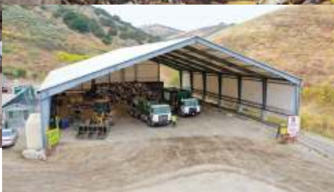
Above: Fabric-clad Truss Arch frames allow for natural lighting with the option of supplemental electric lighting.
