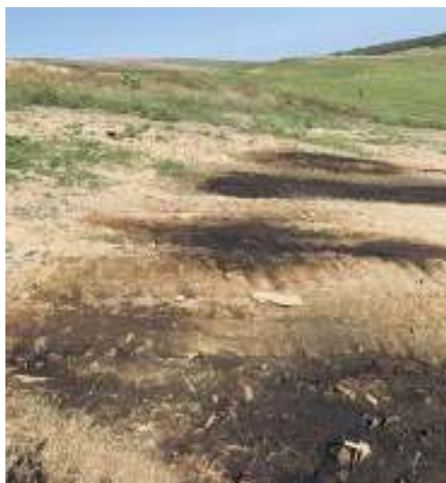
Figure 1: What appear to be shadows in the images are seeps of dark leachate.
